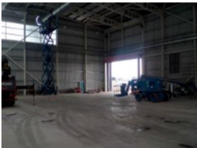
Internal View of Current Progress
