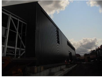
Project During Construction
